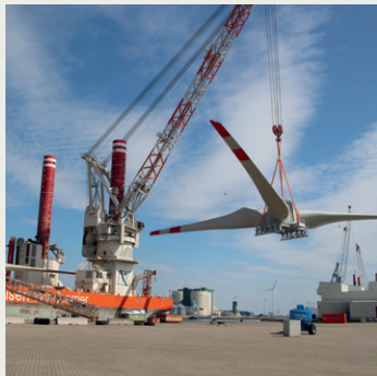
First rotor star lift at Eemshaven
