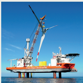
First rotor star installation
