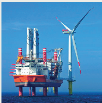
Bold Tern installing a WTG
