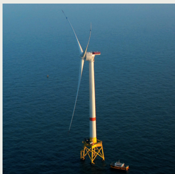
Successful completion of the project
